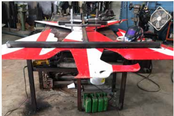
The T-Bird sign sits on metal stands in the Casper College welding shop. New braces were welded to the back of the sign and a new metal post was created to hold the sign and was placed into the cement pillar. (Casper College photo)
